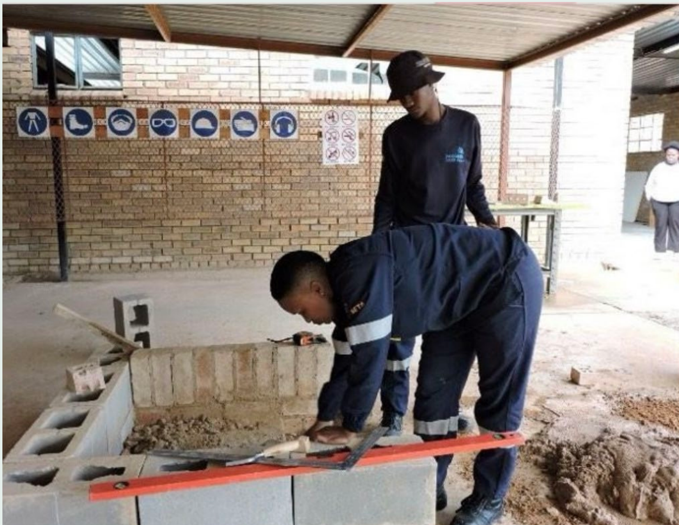
Bricklaying students during the trade test
