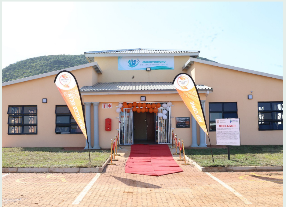
The newly built Mashiyinduku Skills Development Centre in Mange village, Mkuze, KwaZulu-Natal
